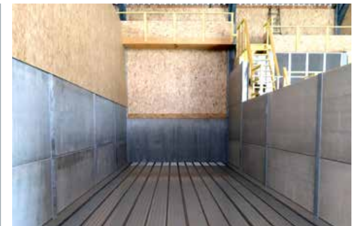
Hay drying system with combined drying floor for drying various bulk materials.
